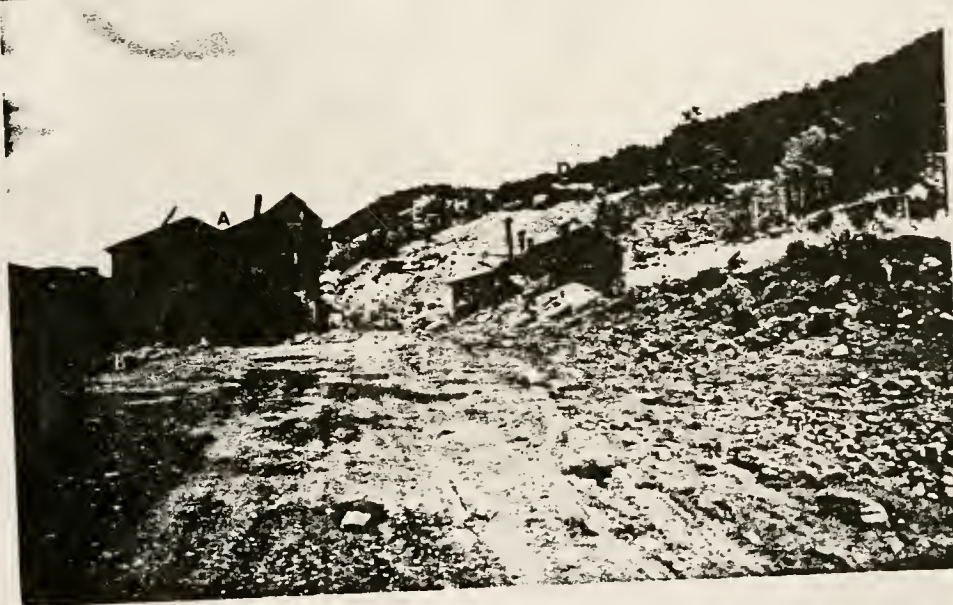
Figure 150. A) Arsenic plant (structure #59) B) Cyanide vats (structure #61) C) Assay office (structure #58) D) Electric substation (structure #54) E) Revenue Mill (Structure #34) (north view)
